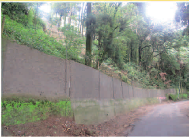
Emergent restoration of landslide
