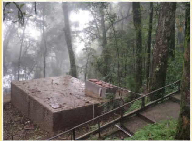
Construction of water reservoir
