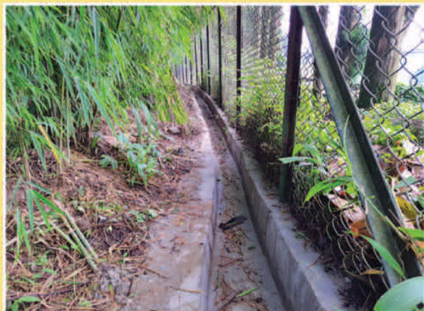
Construction and Repair of drains
