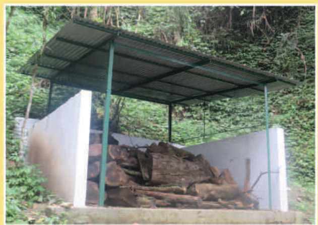
Firewood shade at burning house
