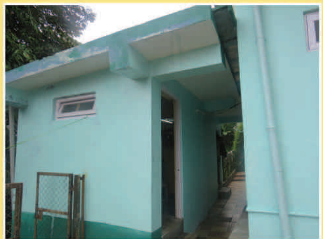
Extension of FRH kitchen
