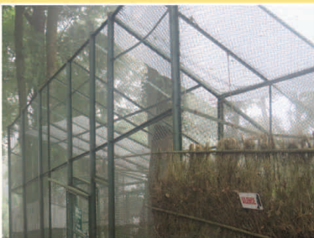
Renovation of Langur enclosure
